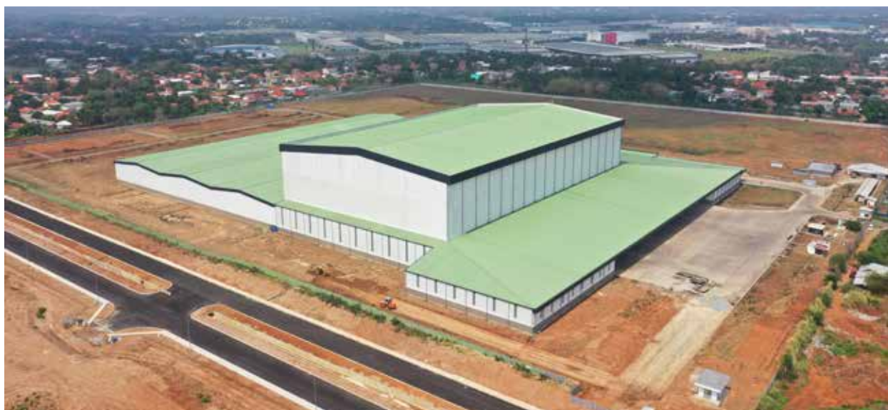
Keterangan foto / Photo caption: Pabrik & Gudang baru Perseroan di MM2100 / New Factory & Warehouse company at MM2100
